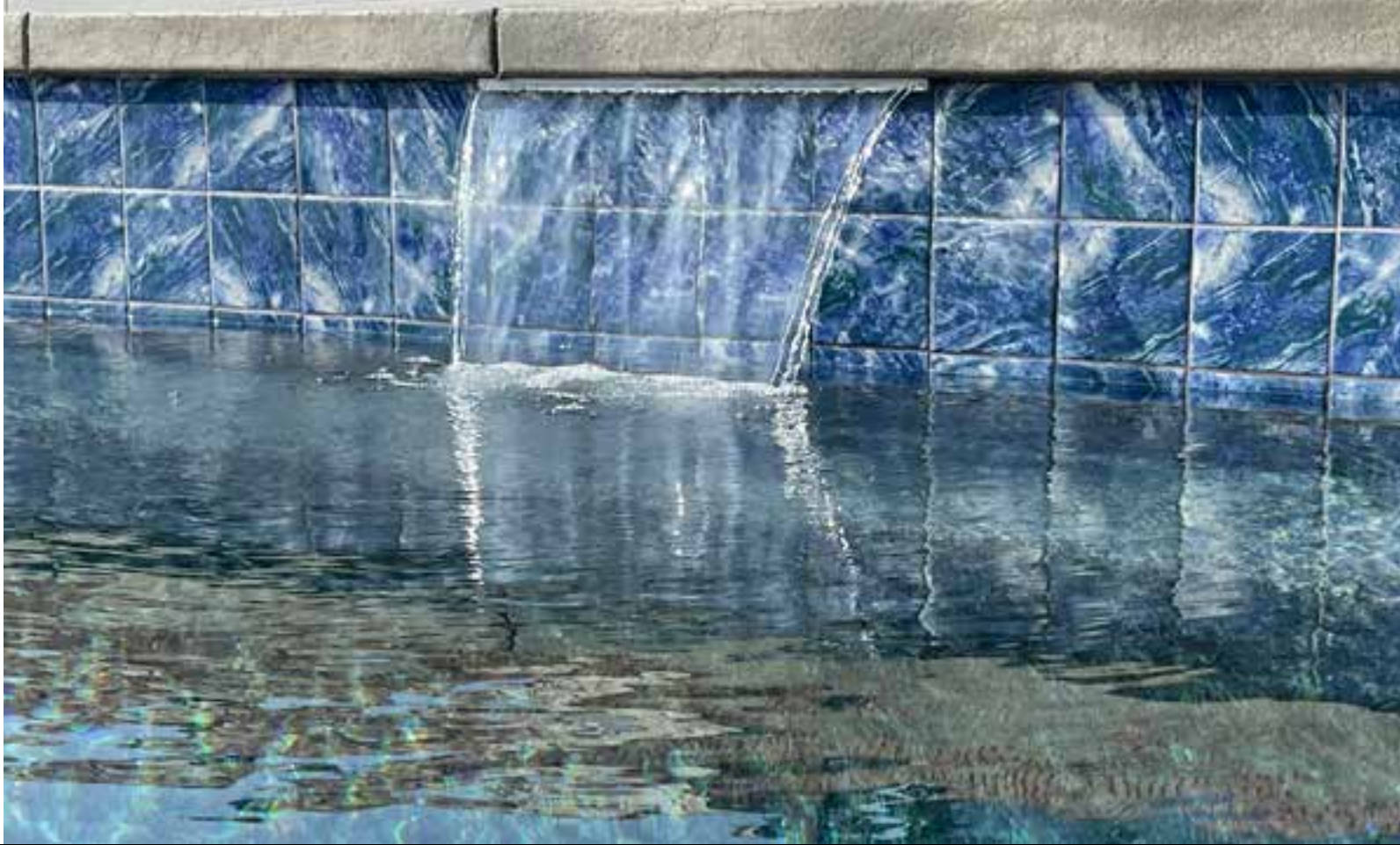
RIO-901 BY QUICKSHOT POOL CONSTRUCTION, CA
